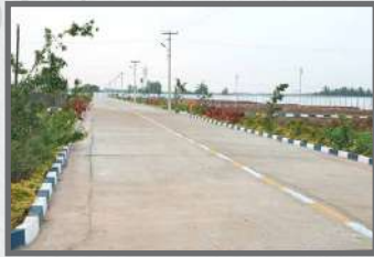
Cement roads with road side RCC drains and footpath.
