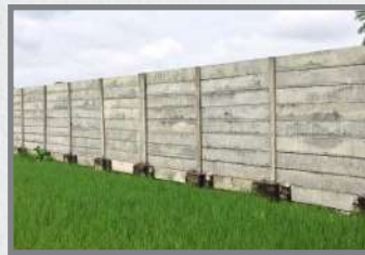
RCC walls Compound.
